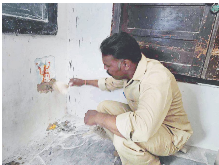
Commencement of 2nd phase on 2nd May 2015
