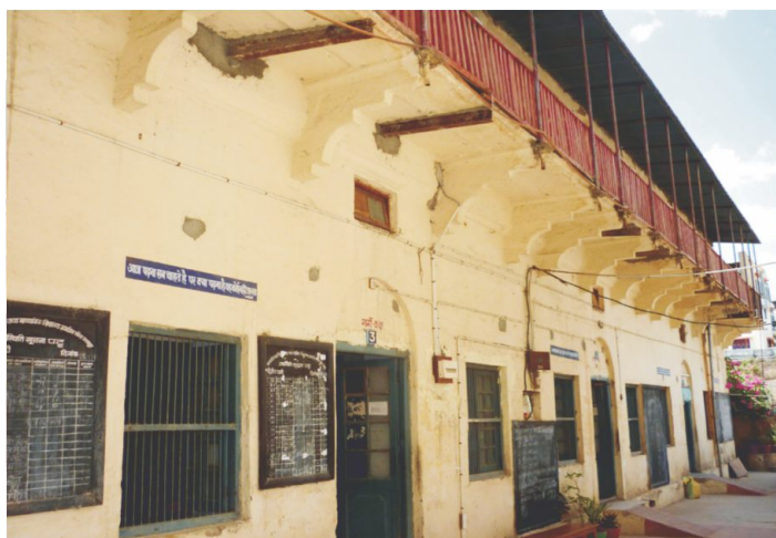
Before (Eastern Facade)
