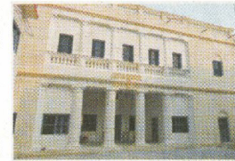
School building after the restoration
