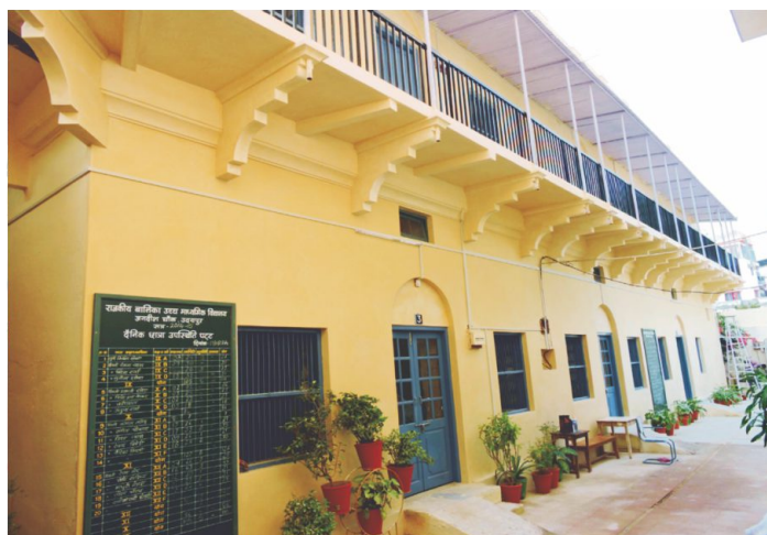
After (Eastern Facade)
