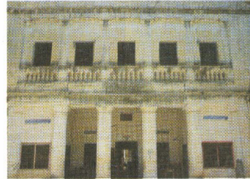
School building before the restoration
