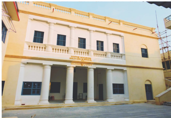
After (Western Facade)
