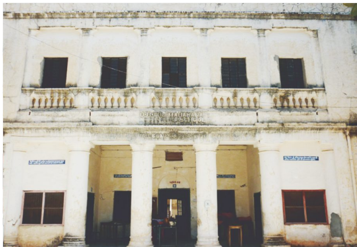
Before (Western Facade)
